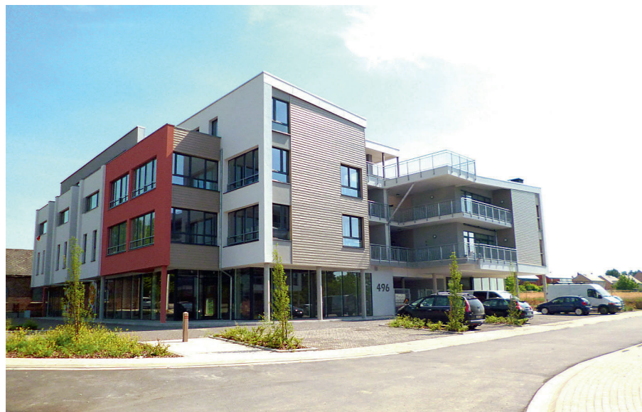
Erpent, Porte Saint-Gerard. Source : thiran.be
